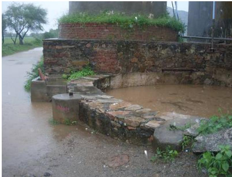
**3. Borunda Village** – A community based approach replicated in Borunda village of Jodhpur district through diverting rainwater run-off channels into 5 deep wells.
